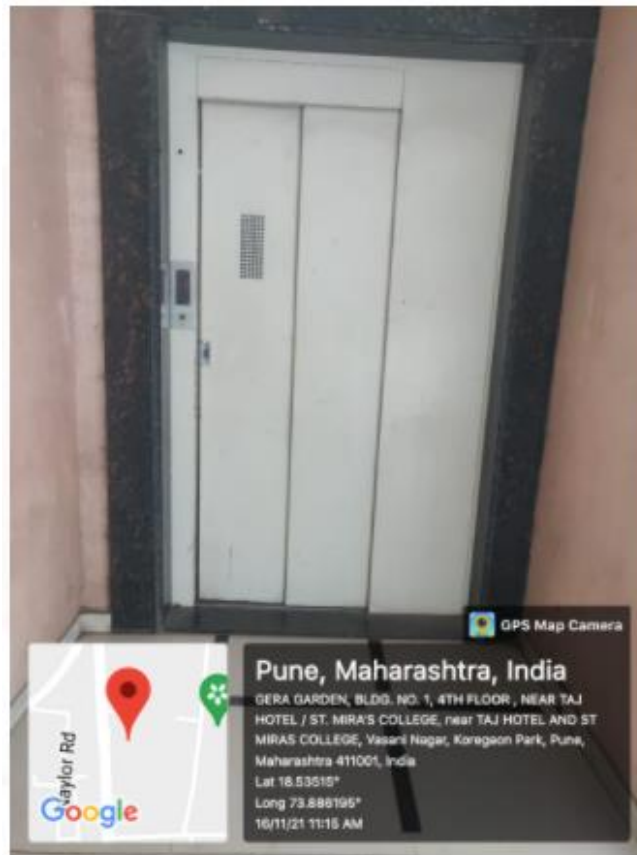
Photo 2 Lift for Specially-abled
